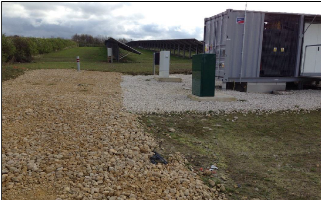
Plate 5: Typical Type 2 Aggregate Solar Farm Track 18
